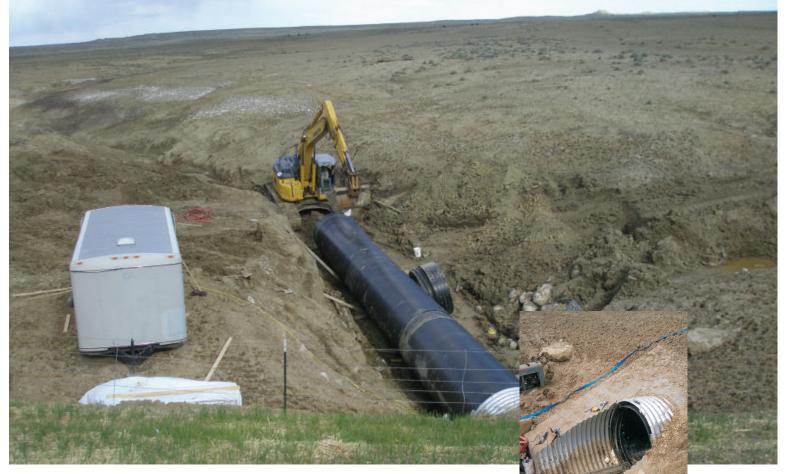
Just south of the Montana State line on Wyoming State Highway 120 north of Cody, the Wyoming Department of Transportation identified a problem with one of their culverts beneath the road. Due to extreme amounts of rainfall and snow runoff, officials were concerned that the road may be compromised if the existing culvert were to fail.
